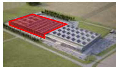
Image of YASKAWA Europe Robotics after expansion (Red area: Robot system plant & ERDC)
