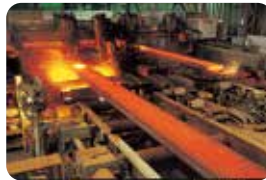
Electrical systems for steel plants
