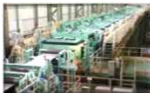
Process line equipment
