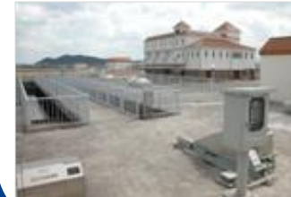
Electrical instrumentation systems for water and sewerage
