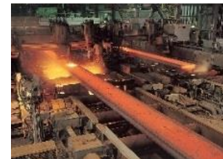
Electrical systems for steel plants
