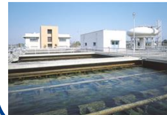
Electrical instrumentation systems for water and sewerage
